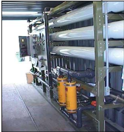
Reverse Osmosis Unit Near Completion
